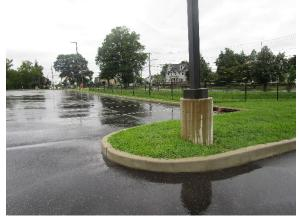
Two sections of pervious pavement parking spaces can be installed at the low side of the parking lots. This will capture and infiltrate parking lot runoff. A preliminary soil assessment suggests that the soils have suitable drainage characteristics for green infrastructure.
